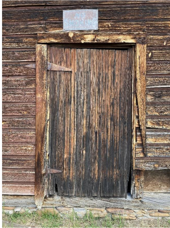
Photograph of representative door on the north elevation, showing door type, casement, and the uncut stone foundation.
