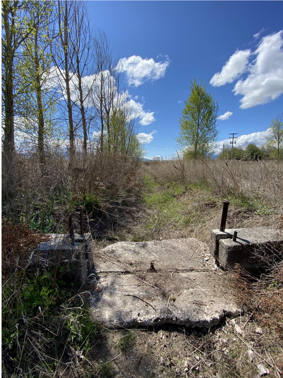
Abandoned headgate structure on the Flynn-Dougherty Ditch (24MO0901) at the Dougherty Ranch, view to the south.
